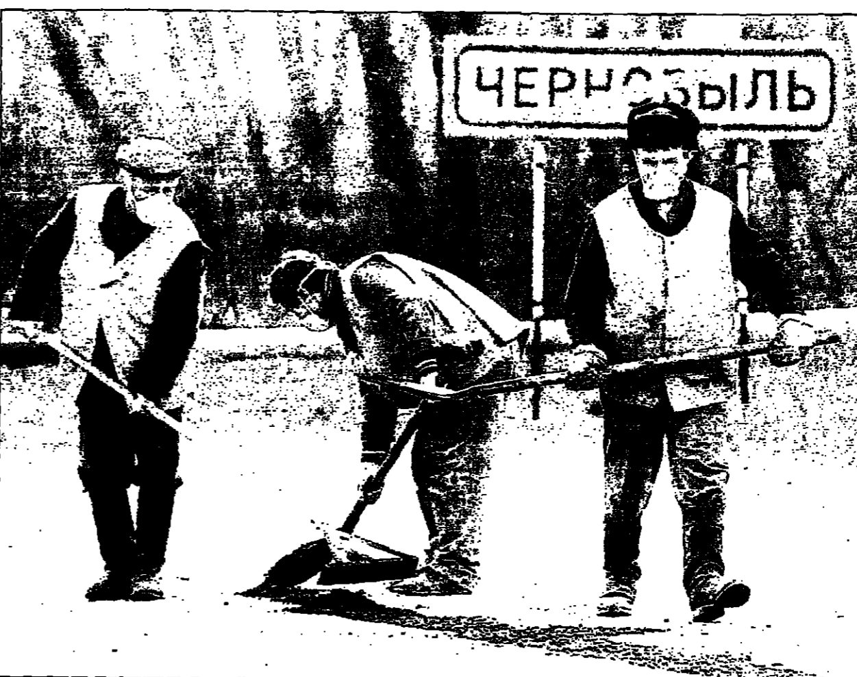
Workers in protective gear repair potholes along a road leading into the town of Chernobyl yesterday
